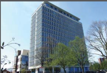
The Heights Bedford 14 Storey Tower of 152 Apartments
